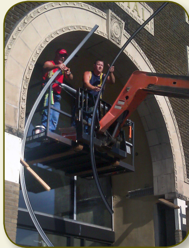
Commercial Glass specialists, Justin and Kevin lift up the finishing pieces of the archway's aluminum frame
